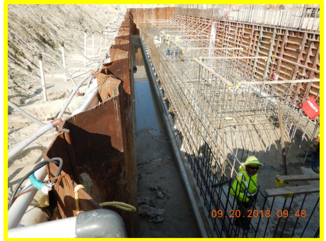
Foundation for Transfer Pump Station
