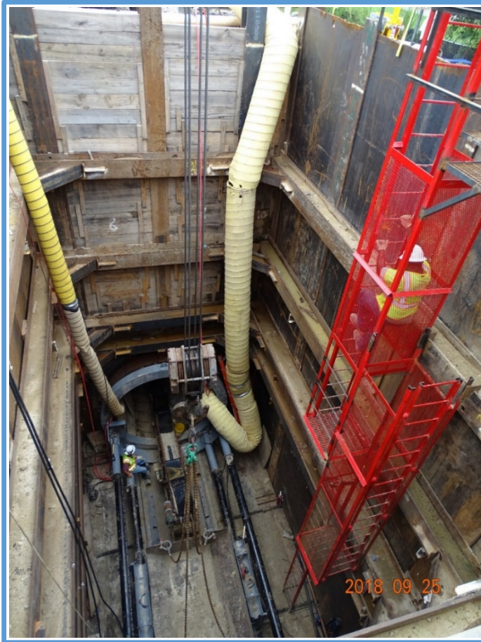
Tunneling under West Lake Houston Parkway is ongoing
